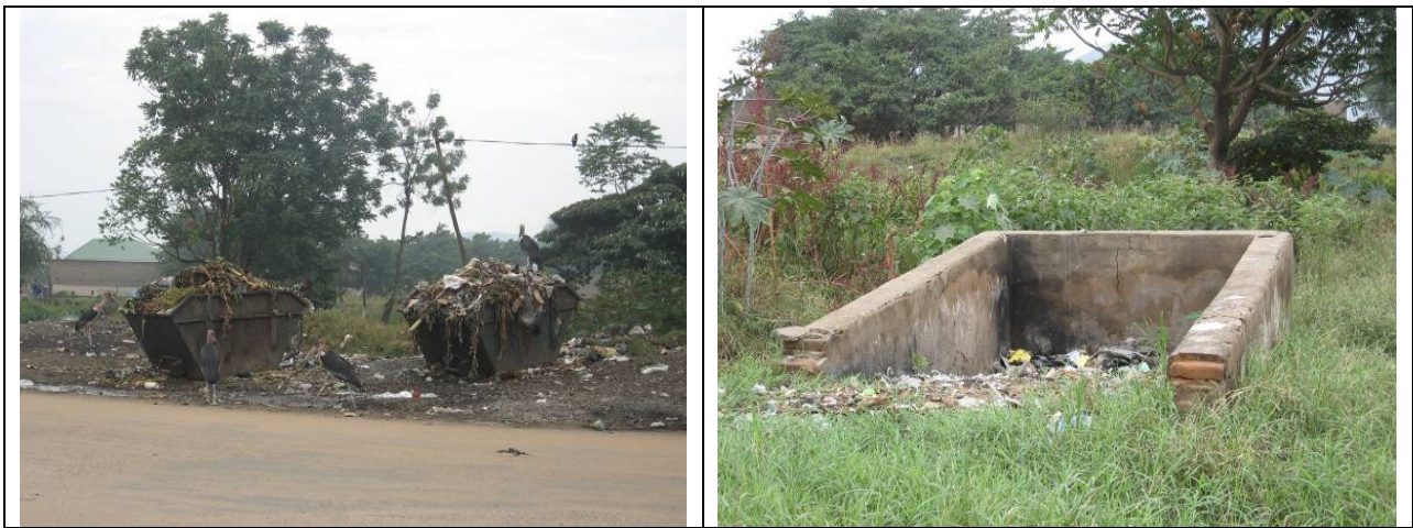
Some of the waste handling infrastructure in Kasese Town Council and their current status
