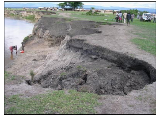
Figure 5: An eroded river bank threatens a village.
