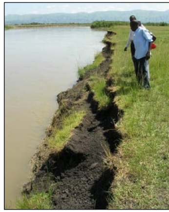
Figure 4: The process of riverbank breakage.
