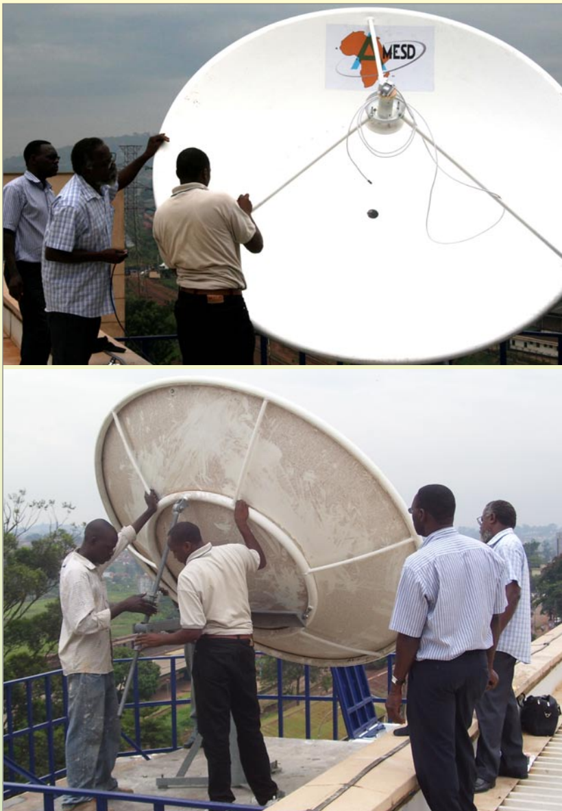
AMSED dish being installed on the rooftop of NEMA House station.
